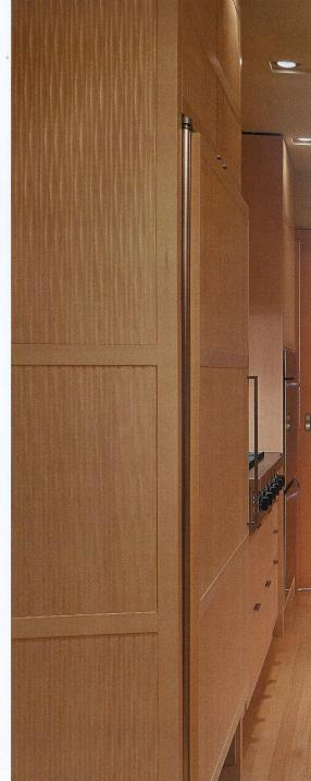
Top left and right, and above right: To screen the dining room, Finne designed an L-shaped pocket door with an interlocking detail on the joint.
